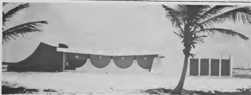
IOWUA's new Recreation Center on the Boulevard inaugurated August 10.
